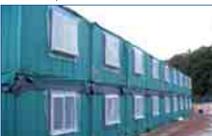
Modular building - Officers' single living accommodation
