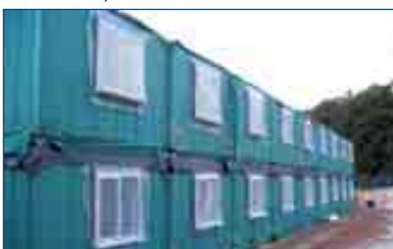
Modular building - Officers' single living accommodation
