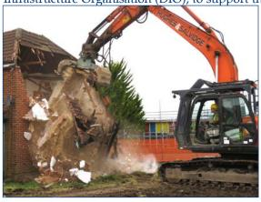
majority of materials recovered from demolitions, such as bricks, timber joists and métal, are removed from site to be reused or recycled, mińimising waste sent to landfill.
